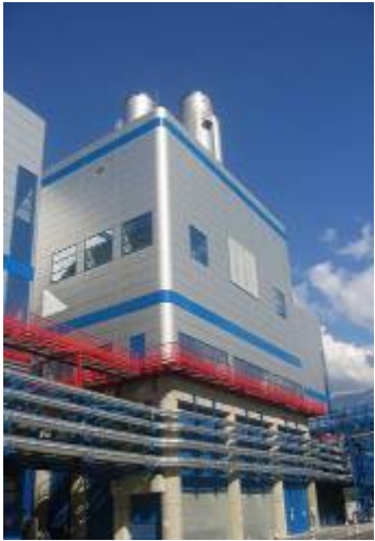
Process exhausts 580 000 m 3 /h
